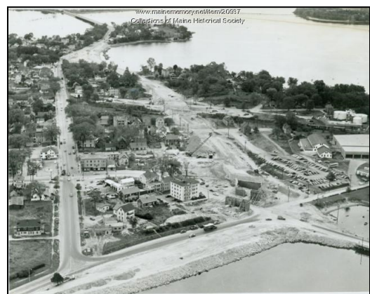
Figure 4. Work on the East Deering I-295 Bypass in 1953 which separated the neighborhood from the coast (looking northeast). Source: Maine Memory Network
